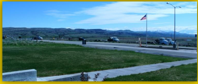
Repaving the Front of Logan's Entrance
