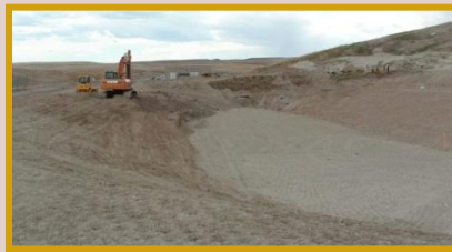
Logan Landfill crew working on the old leachate pond, preparing it for the new improvements approved by MDEQ.
