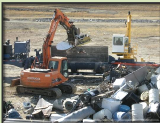
Metal Scrap being processed by contractor for market
